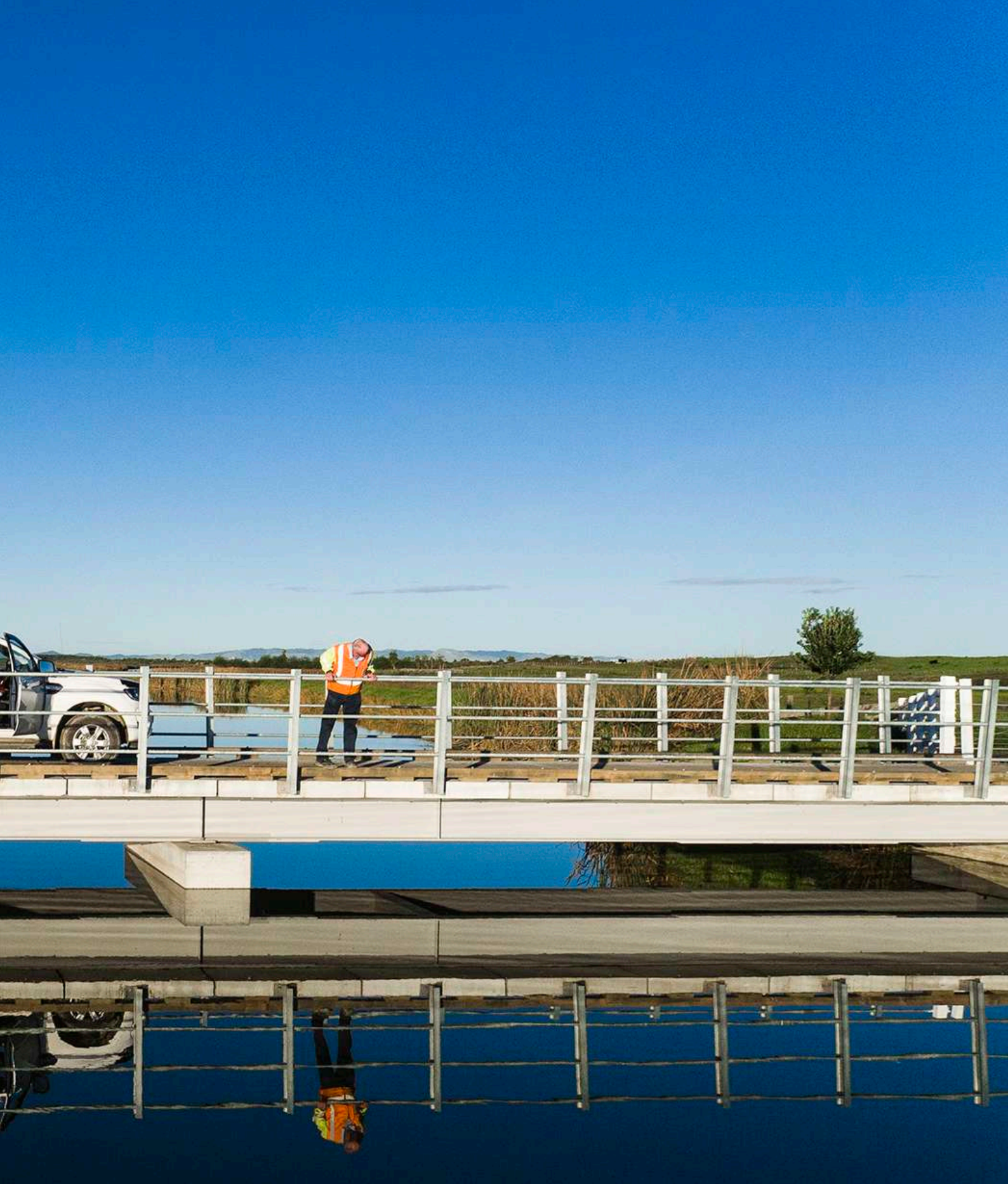
The new class 2 Patangata Bridge crosses Rahui Channel 14km east of Wairoa at Whakakī. The bridge, which was backed by the Provincial Growth Fund, is essential for people to safely access land and urupā (burial grounds) across the channel. Lattey Group prefabricated the deck and handrails offsite, and the abutments and pier onsite. An 80-tonne heavy lift crane was used for assembly while QRS completed the roading approaches and erosion control.
